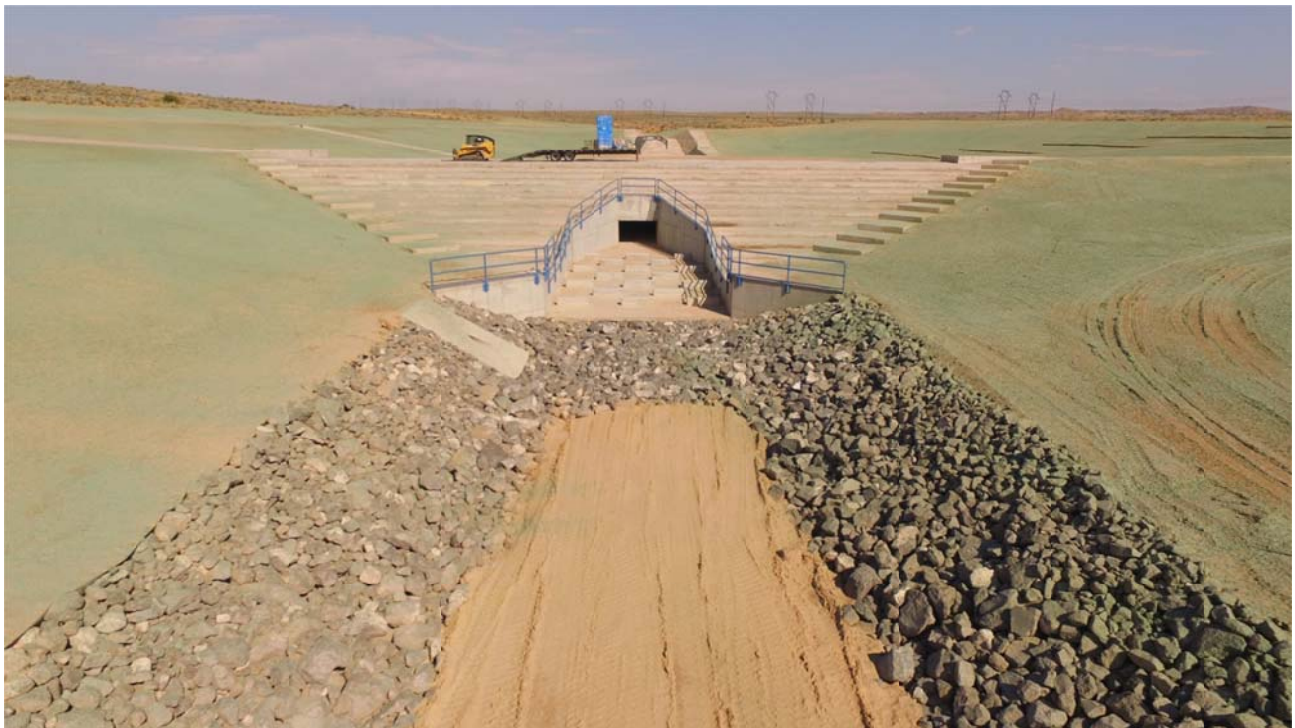
Southern Sandoval County Arroyo Flood Control Upper SLO Dam Construction
