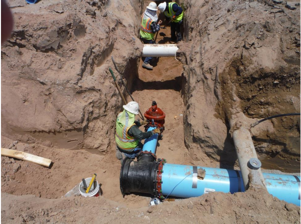
Doña Ana MDWCA Inter-connecting water systems - extending waterlines to serve additional residents
